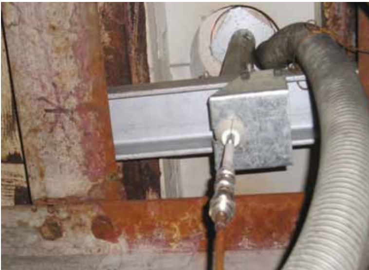
Bubbler block over-coat tile supported in position.
